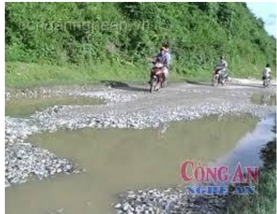
Fig. 7 Road pavement damage
