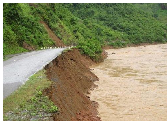
Fig. 8 Land slide of the slope
