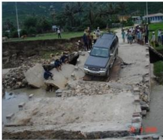
Fig. 5 Damage of pier lead to bridge collapse
