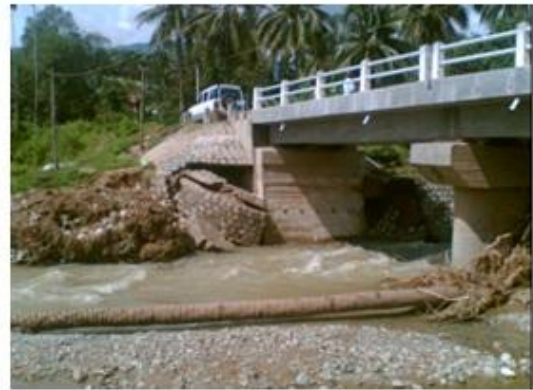
Fig. 3 A Flood in Ha Tinh (2003) damage the abutment of a bridge
