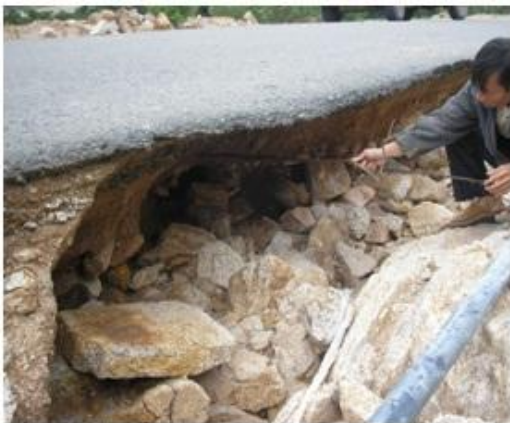
Fig. 6 Erosion of roadbed
